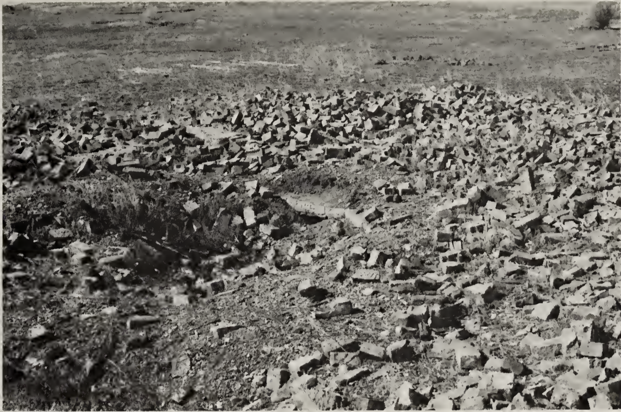
Figure 41: Central Pacific shop & office building (BLM photo)
